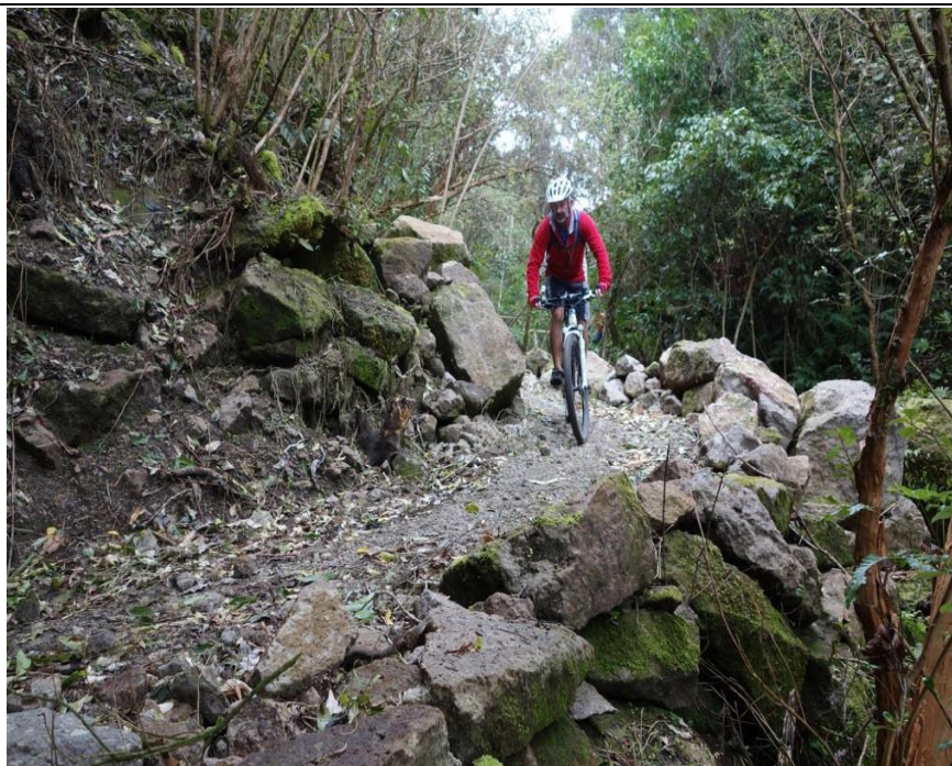
Figure D10: Rock armoured path – Nichols Creek Track, Dunedin (Photo: Kennett Brothers)
