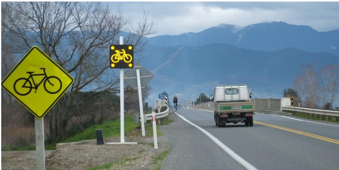
Figure 26: Inductive loop activated warning sign on Appleby bridge, SH 60, near Nelson (Photo: NZTA)
