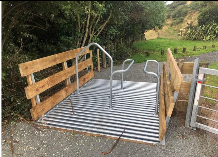
Figure F14: Example of a wheelchair-accessible barrier, Belmont Regional Park (Photo: Greater Wellington Regional Council)
