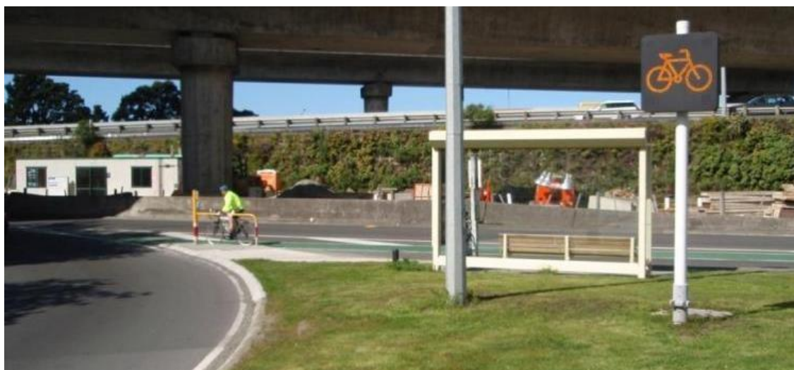
Figure 27: Active warning sign at Ngauranga interchange, SH 2, Wellington (Photo: NZTA)
