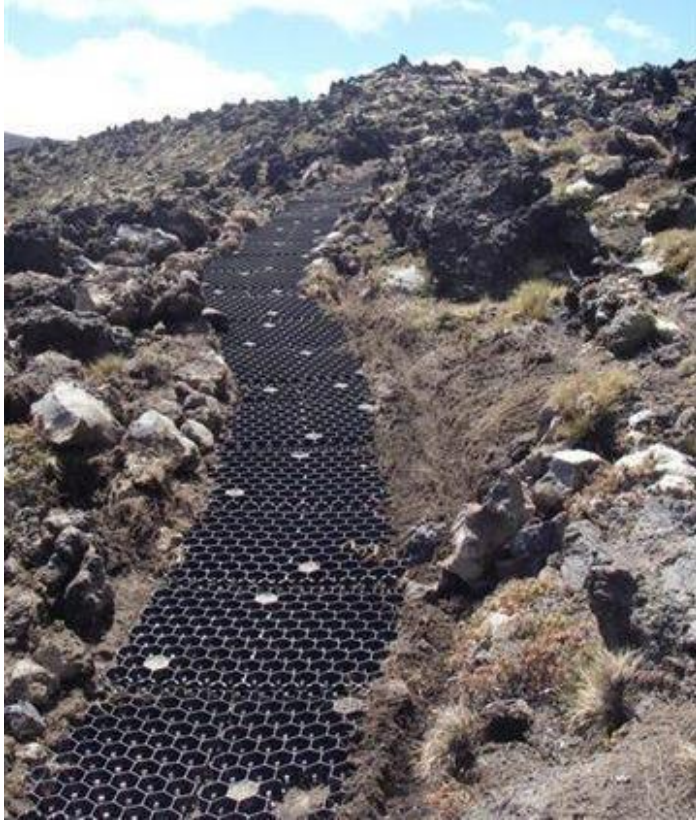
Figure C9: ‘Geomat’ surface stabilisers (prior to having aggregate placed on top), Tongariro National Park (Photo: John Bradley)
