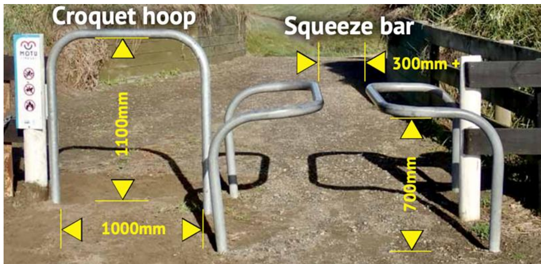
Figure C11: Accessibility modifications for hoop and squeeze barriers
