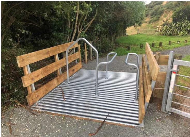
Figure E14: Example of a wheelchair-accessible barrier, Belmont Regional Park (Photo: Greater Wellington Regional Council)
