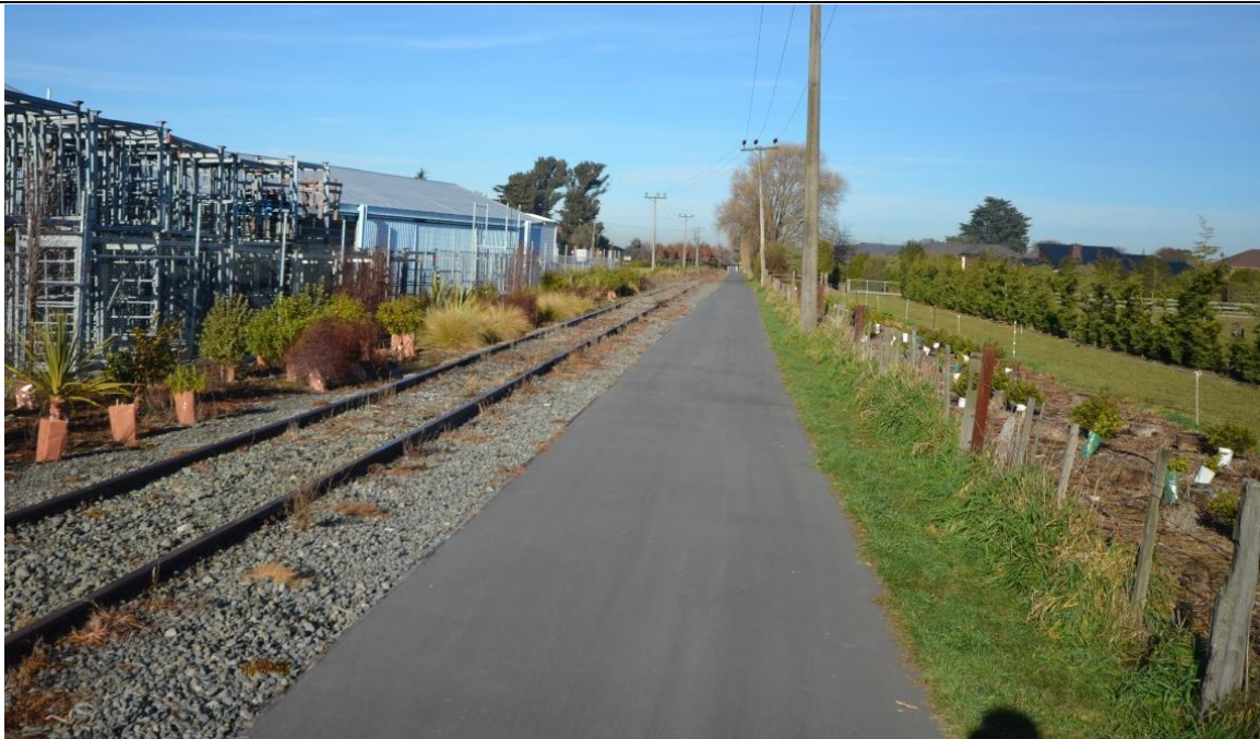
Figure B12: Asphaltic concrete path on the Little River Rail Trail (Photo: Jonathan Kennett)
