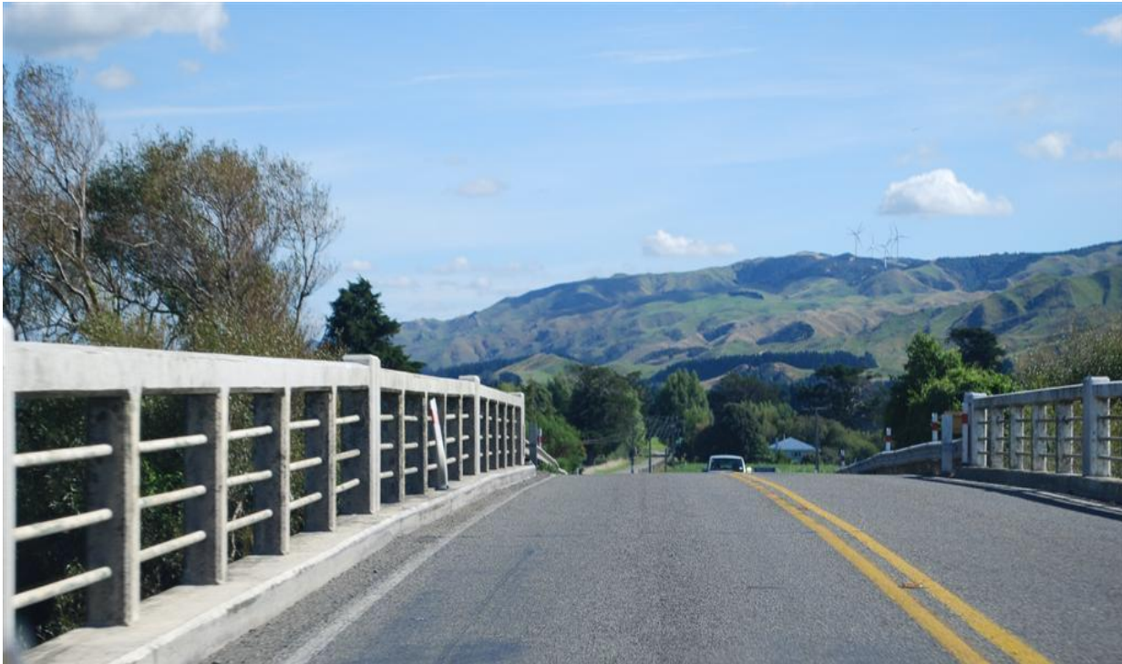
Figure 35: Many railway over-bridges have inadequate shoulder width and may require clip-on bridges on each side for cycling safety (Photo: Jonathan Kennett)
