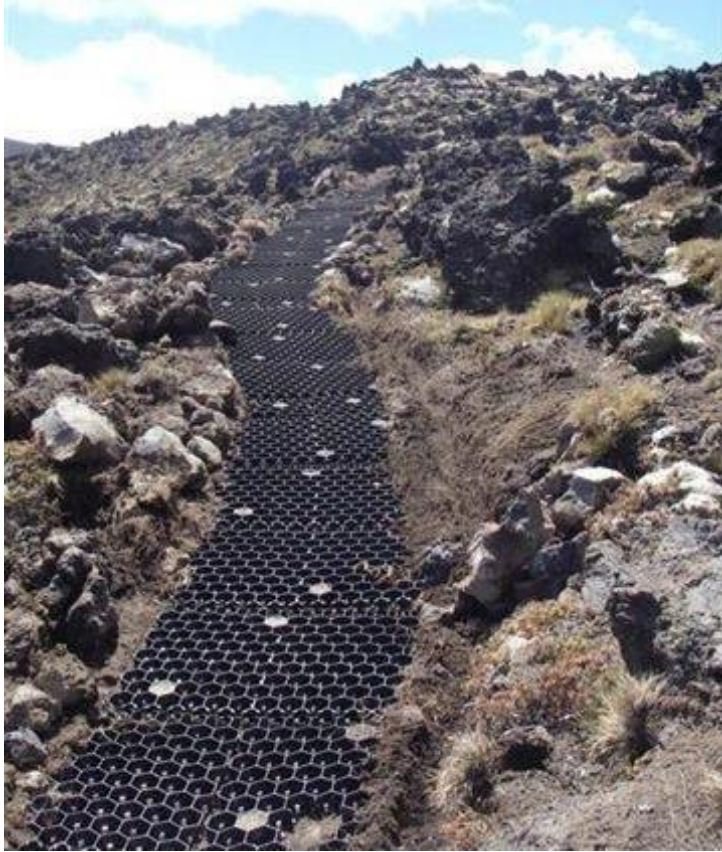
Figure D9: 'Geomat' surface stabilisers (prior to having aggregate placed on top), Tongariro National Park (Photo: John Bradley)
