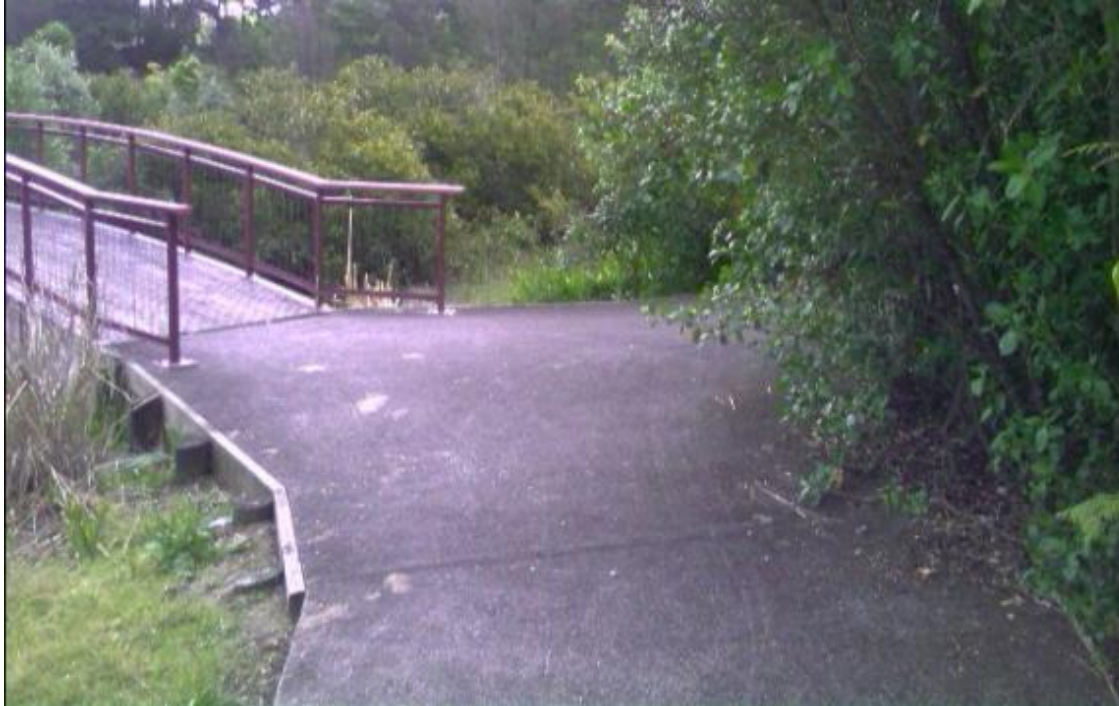
Figure 33: Poor inter-visibility at path intersection – Auckland
