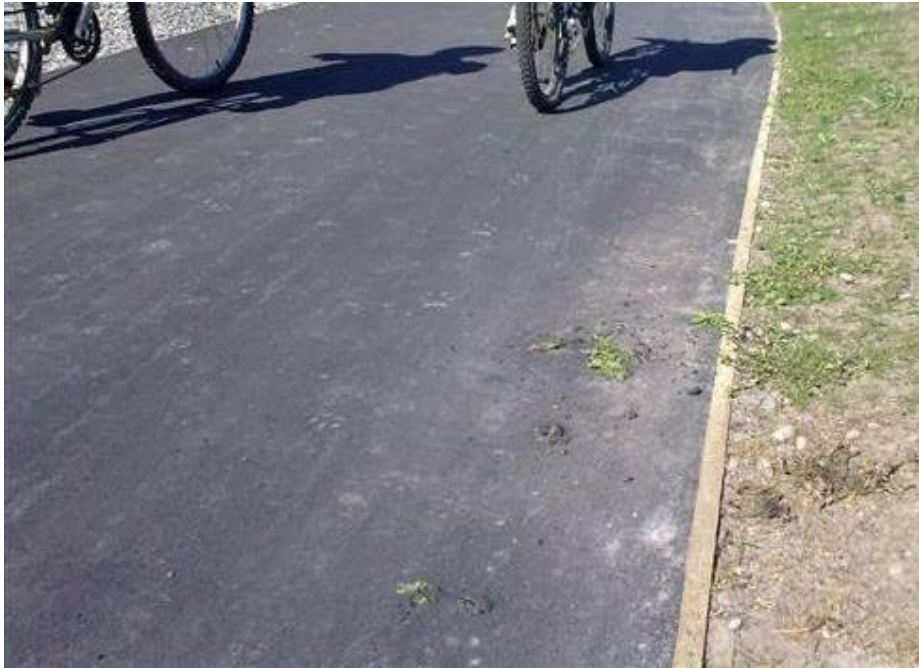
Figure 78: Vegetation growing through new asphaltic concrete path; good construction specifications and contract supervision are required
