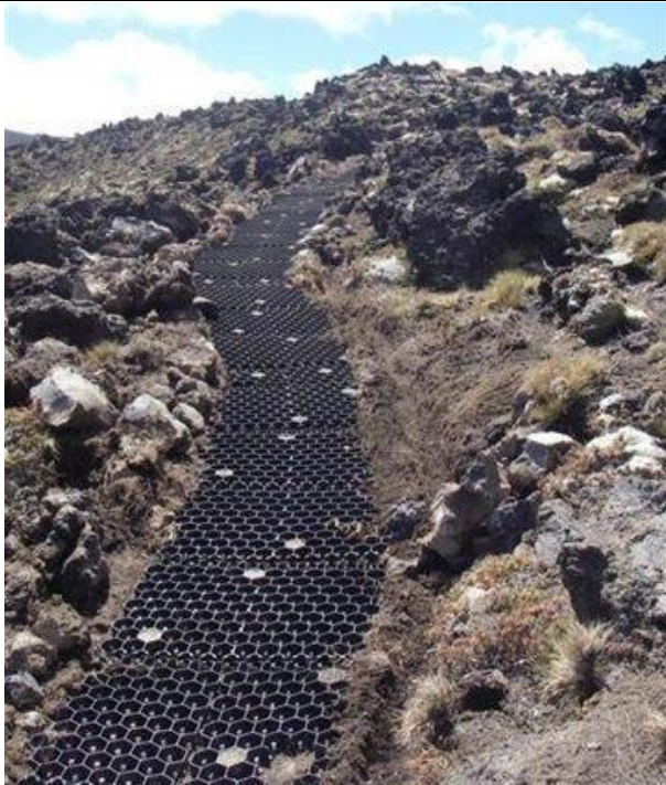
Figure B8: 'Geomat' surface stabilisers (prior to having aggregate placed on top), Tongariro National Park (Photo: John Bradley)
