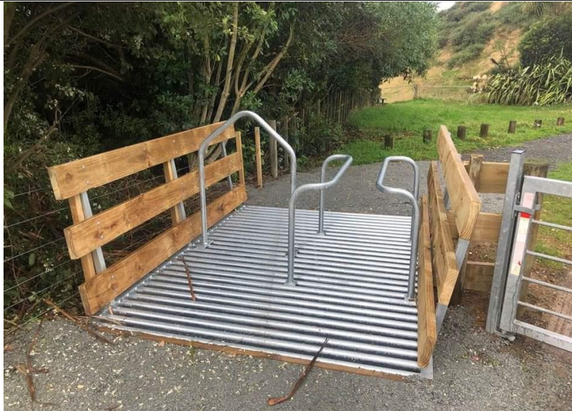
Figure C14: Example of a wheelchair-accessible barrier, Belmont Regional Park (Photo: Greater Wellington Regional Council)
