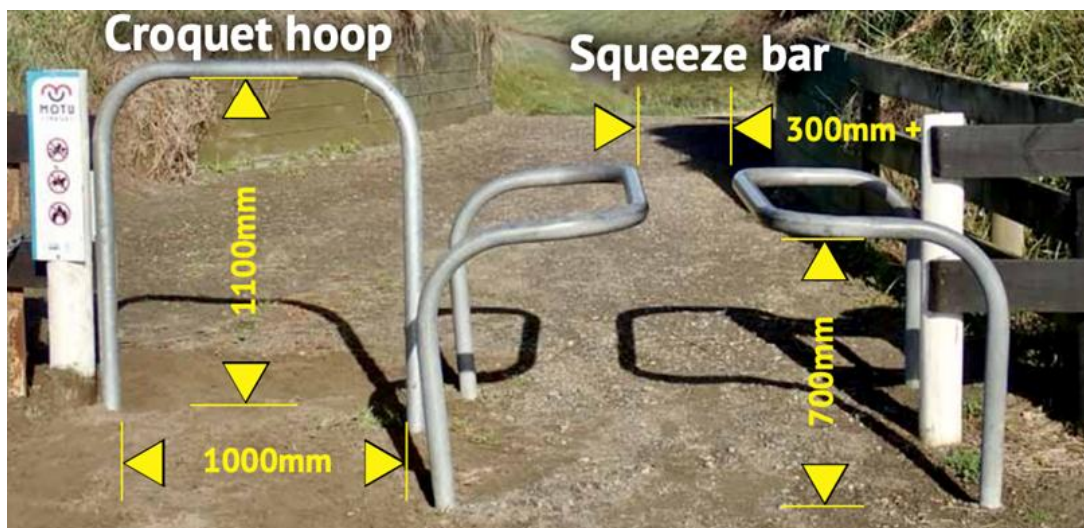
Figure A15: Accessibility modifications for hoop and squeeze barriers
