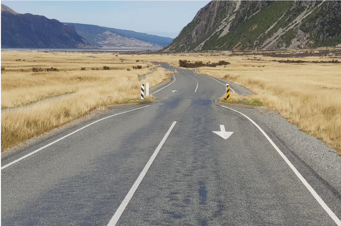
Figure 18: An example of rural traffic calming on a 60km/h road, Hooker Valley
