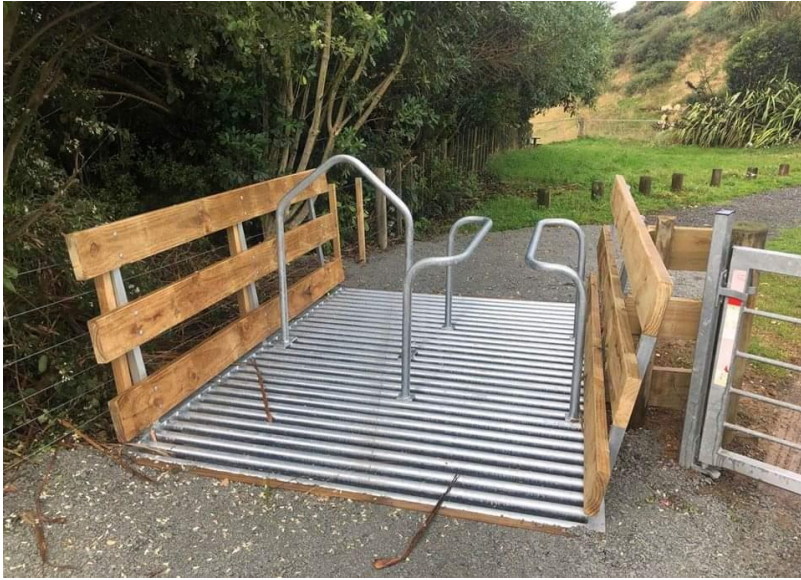
Figure D14: Example of a wheelchair-accessible barrier, Belmont Regional Park (Photo: Greater Wellington Regional Council)
