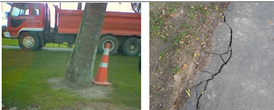
Figure B11: Heavy truck causing edge break on new pathway during construction
