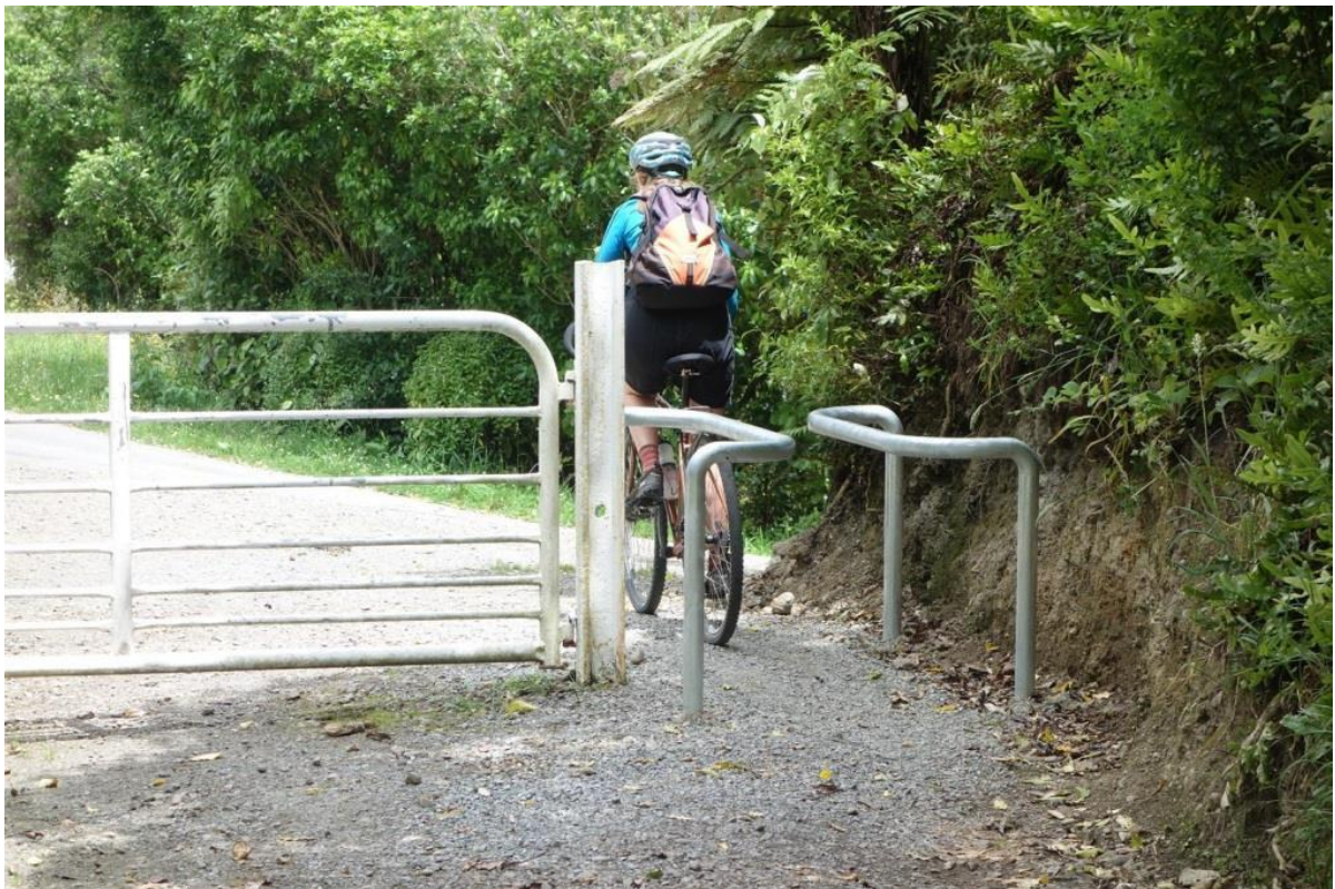
Figure B20: 'Squeeze barrier' to discourage motorcycles, Remutaka Cycle Trail (Photo: Jonathan Kennett)
