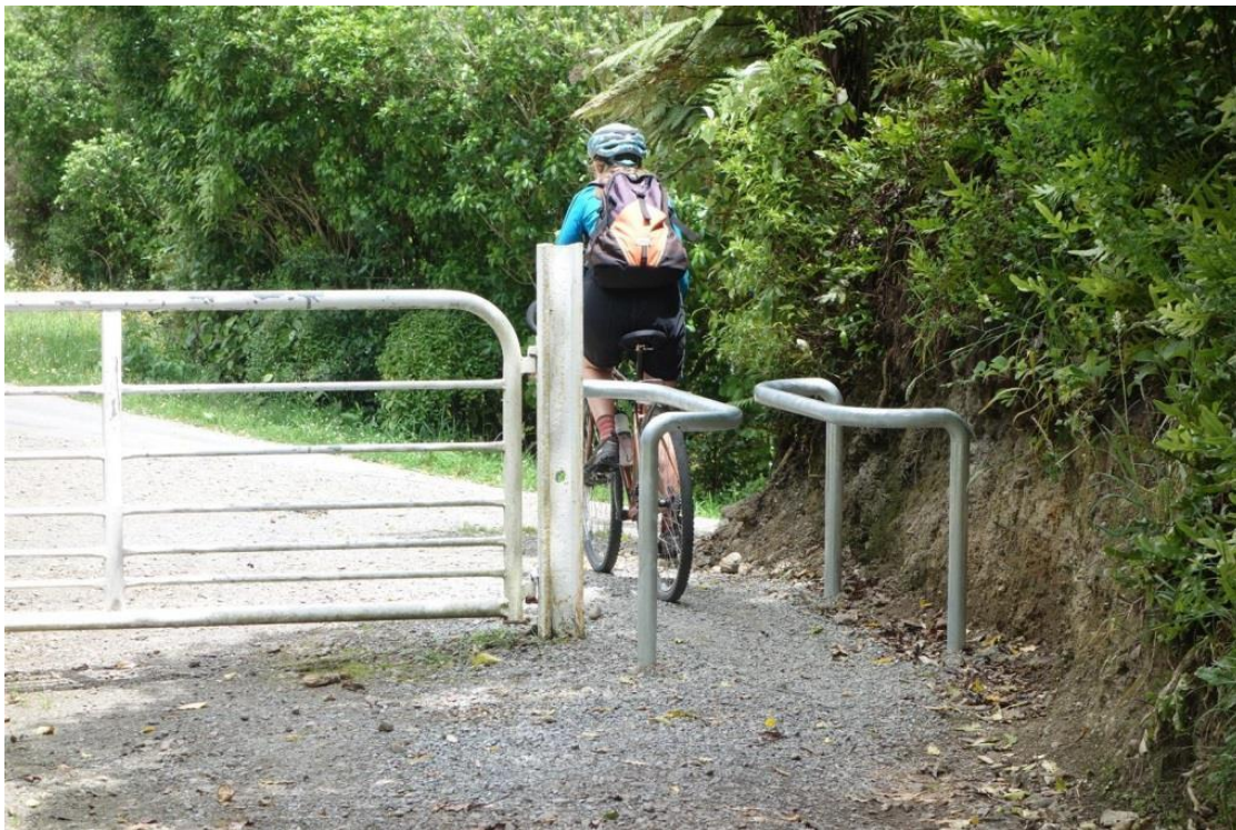
Figure A20: ‘Squeeze barrier’ to discourage motorcycles, Remutaka Cycle Trail (Photo: Jonathan Kennett)
