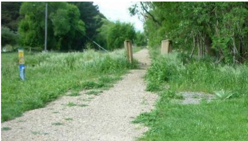
Figure F7: Compacted gravel section of Little River Rail Trail at Catons Bay
