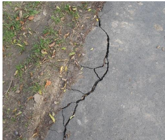
Figure A11: Heavy truck causing edge break on new pathway during construction
