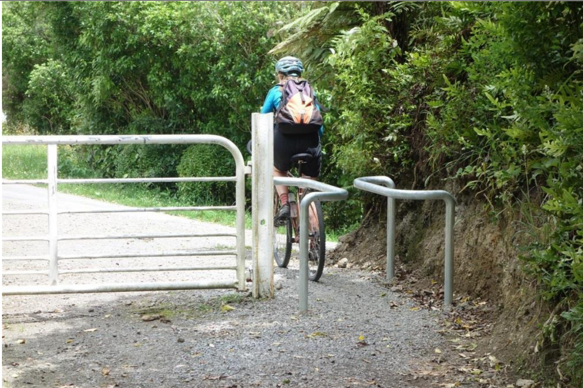
Figure F17: 'Squeeze barrier' to discourage motorcycles, Remutaka Cycle Trail (Photo: Jonathan Kennett)
