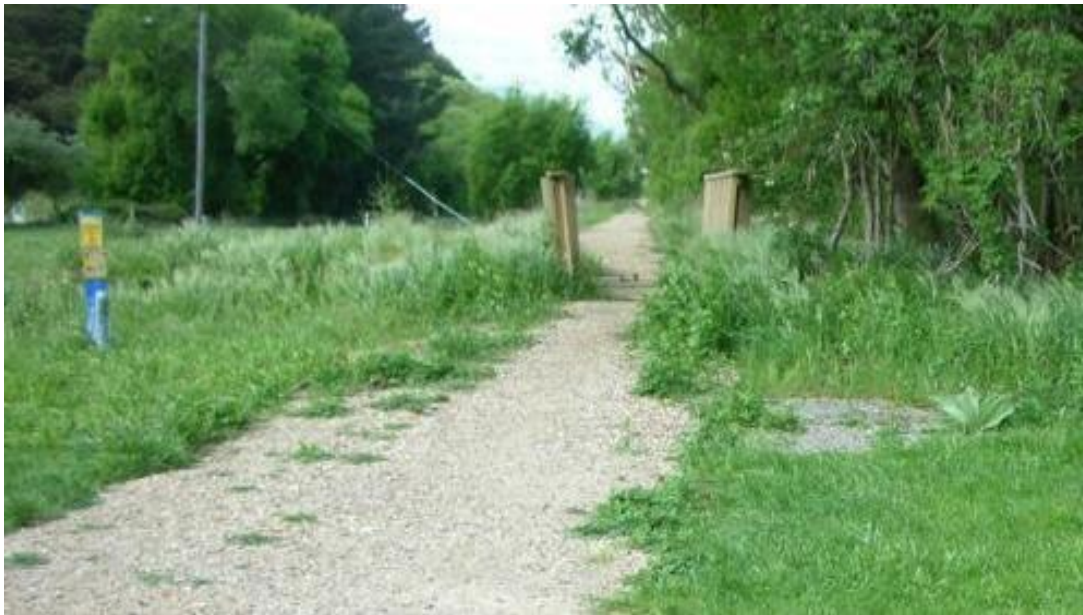
Figure A7: Compacted gravel section of Little River Rail Trail at Catons Bay
