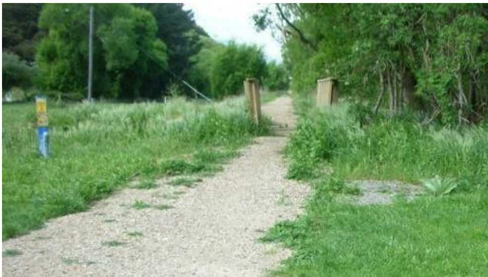
Figure D7: Compacted gravel section of Little River Rail Trail at Catons Bay
