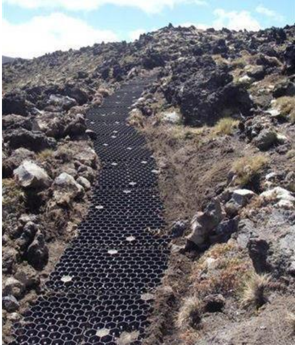
Figure E9: 'Geomat' surface stabilisers (prior to having aggregate placed on top), Tongariro National Park (Photo: John Bradley)
