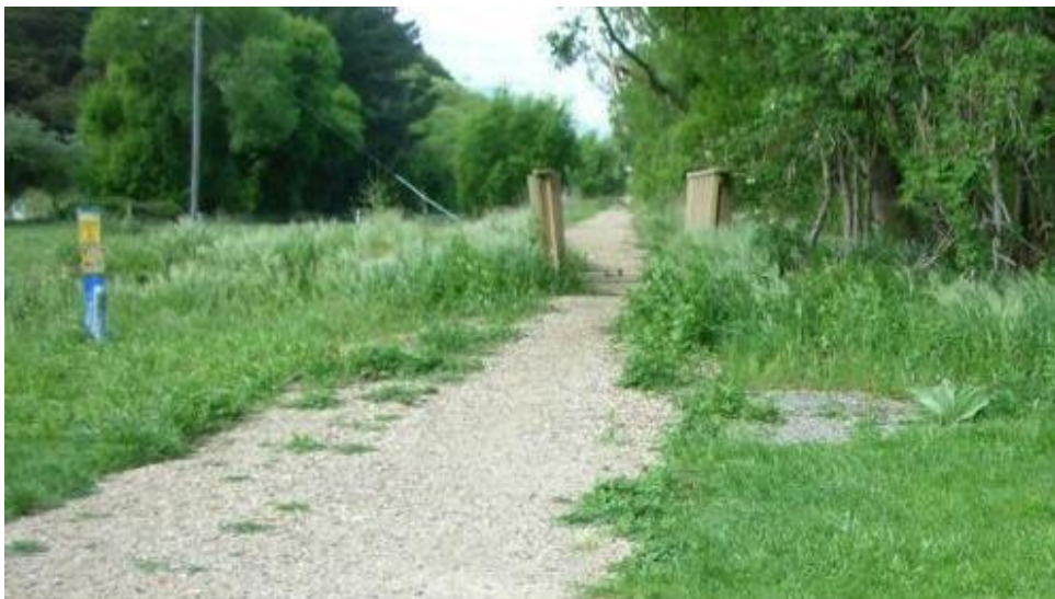
Figure E7: Compacted gravel section of Little River Rail Trail at Catons Bay
