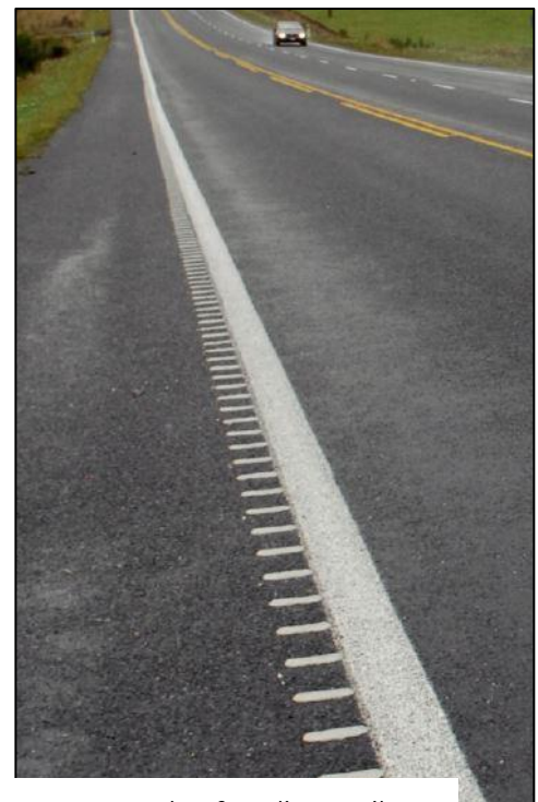
Figure 29: Example of audio-tactile profile (ATP) markings outside an edge-line
