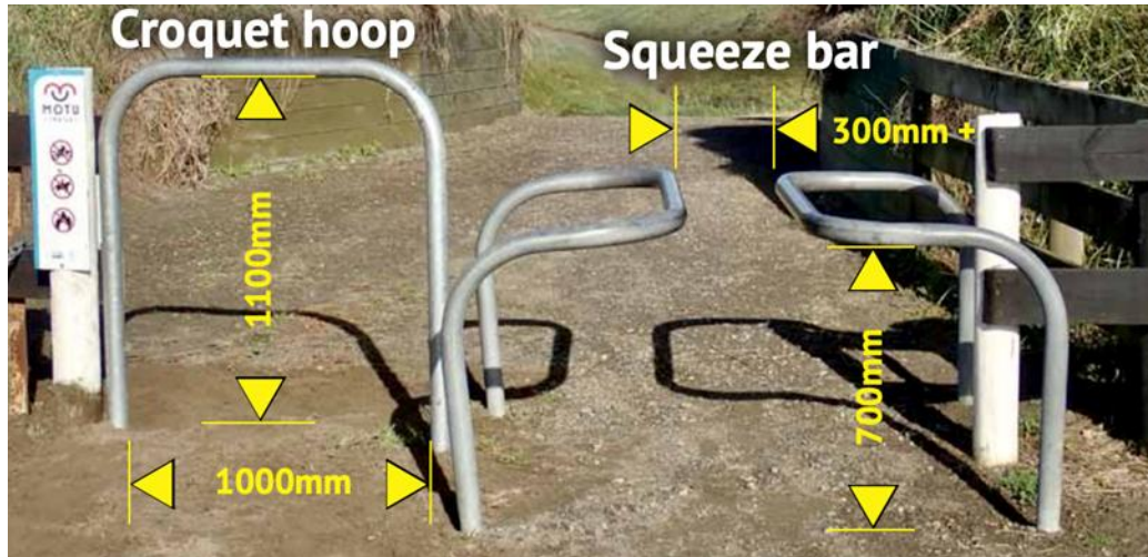
Figure E11: Accessibility modifications for hoop and squeeze barriers
