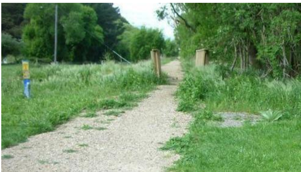
Figure C7: Compacted gravel section of Little River Rail Trail at Catons Bay
