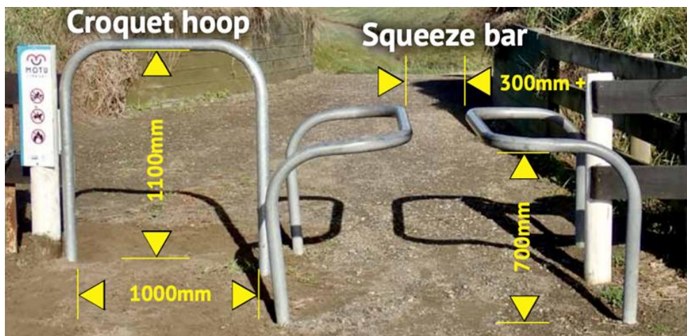
Figure B15: Accessibility modifications for hoop and squeeze barriers
