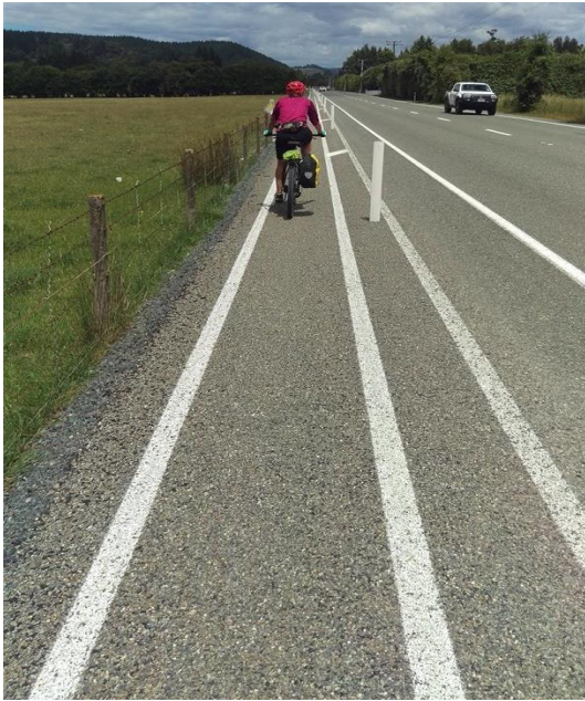
Figure 22: Separated shoulder for contra-flow cycling, SH6 near Wakefield (Photo: Miro Kennett)
