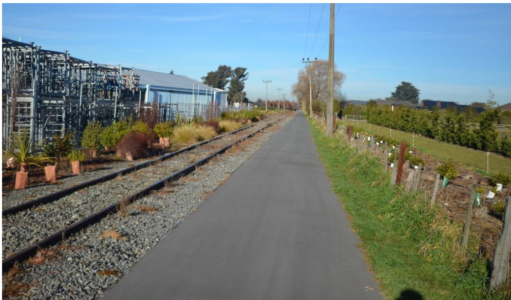
Figure A12: Asphaltic concrete path on the Little River Rail Trail (Photo: Jonathan Kennett)
