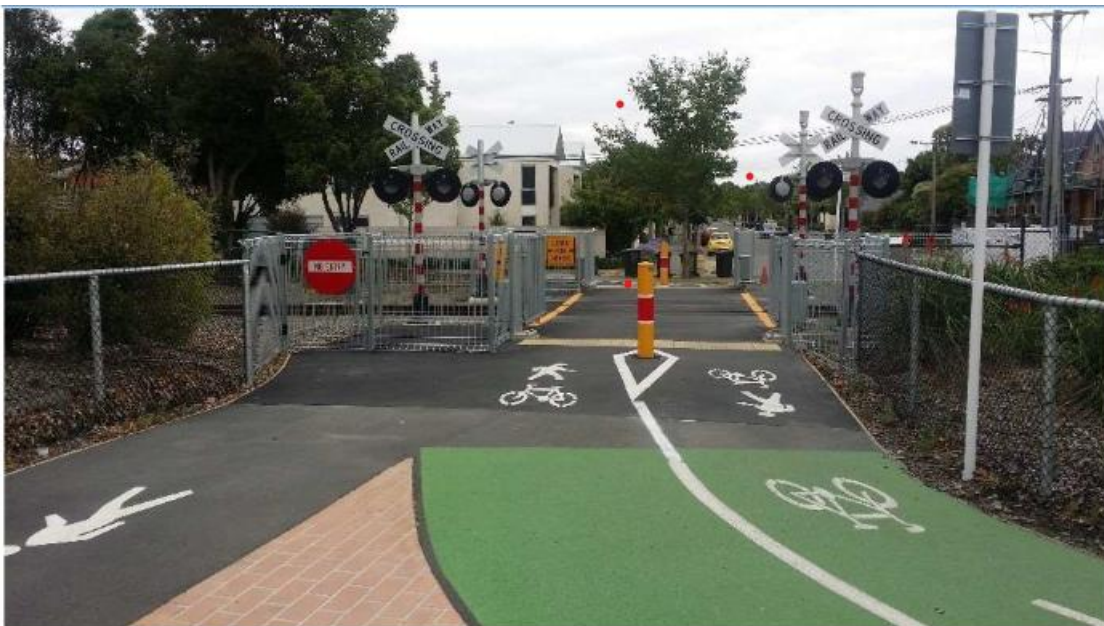
Figure A14: Transition between shared path, footpath and separated cycleway, Matai Street, Christchurch
