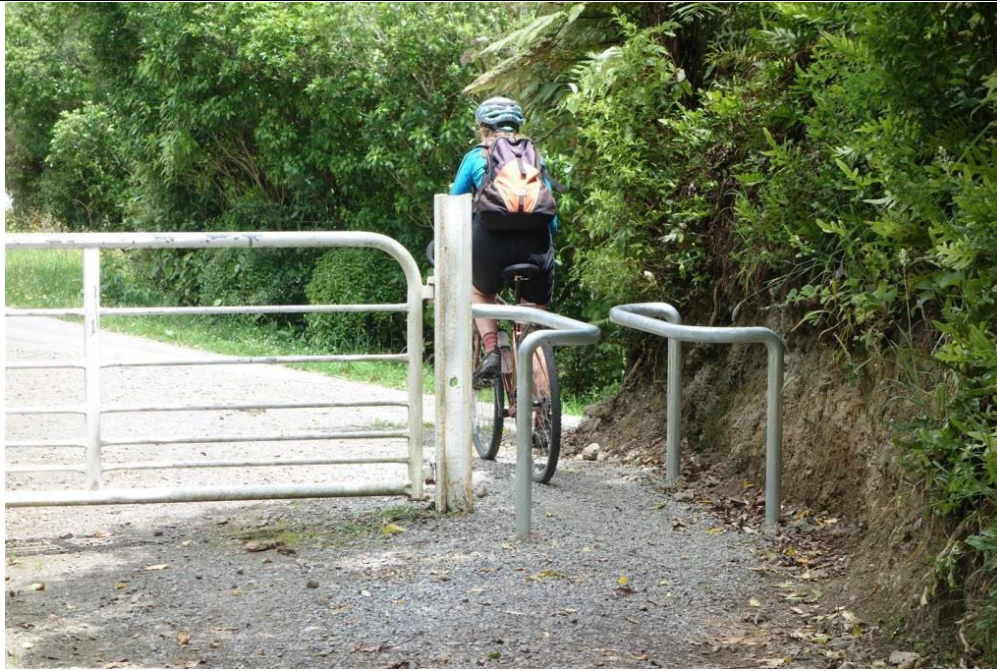
Figure C17: 'Squeeze barrier' to discourage motorcycles, Remutaka Cycle Trail (Photo: Jonathan Kennett)
