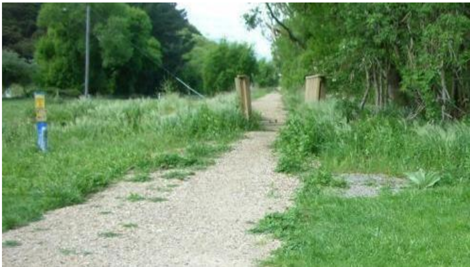
Figure B7: Compacted gravel section of Little River Rail Trail at Catons Bay
