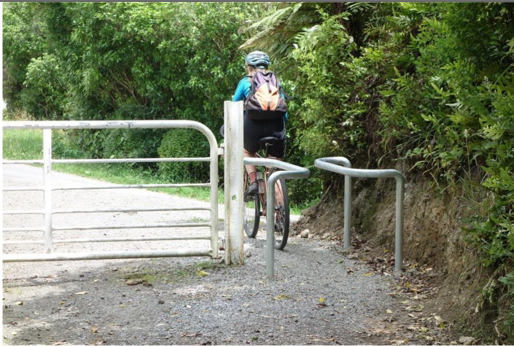
Figure D17: 'Squeeze barrier' to discourage motorcycles, Remutaka Cycle Trail (Photo: Jonathan Kennett)
