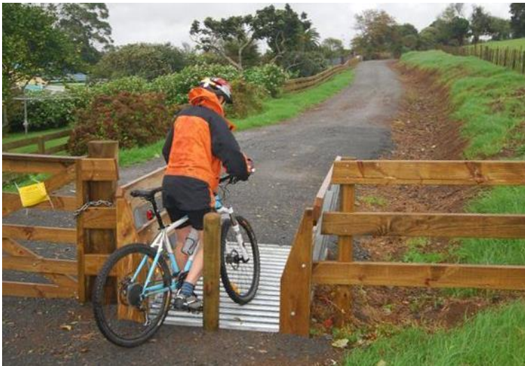
Figure 42: A central post and wing barriers help prevent motorcycle access and reduce the likelihood of stock jumping the cattle stop, but hinder accessibility for cyclists with adapted bikes or panniers (Photo: Jonathan Kennett)
