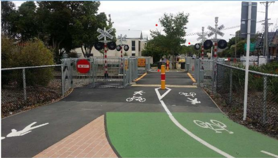
Figure B14: Transition between shared path, footpath and separated cycleway, Matai Street, Christchurch
