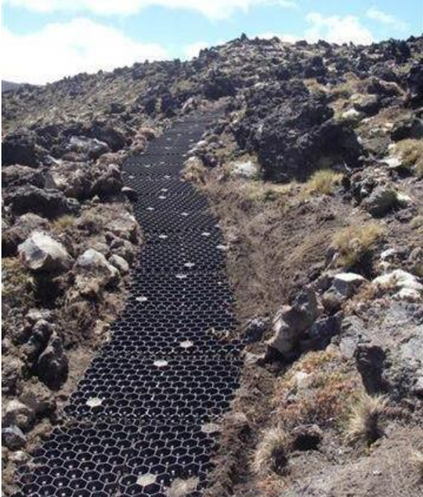
Figure F9: 'Geomat' surface stabilisers (prior to having aggregate placed on top), Tongariro National Park (Photo: John Bradley)
