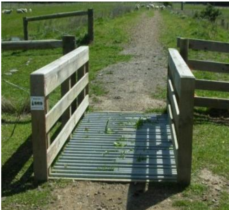
Figure 38: Cattle stop placed on straight alignment of track
