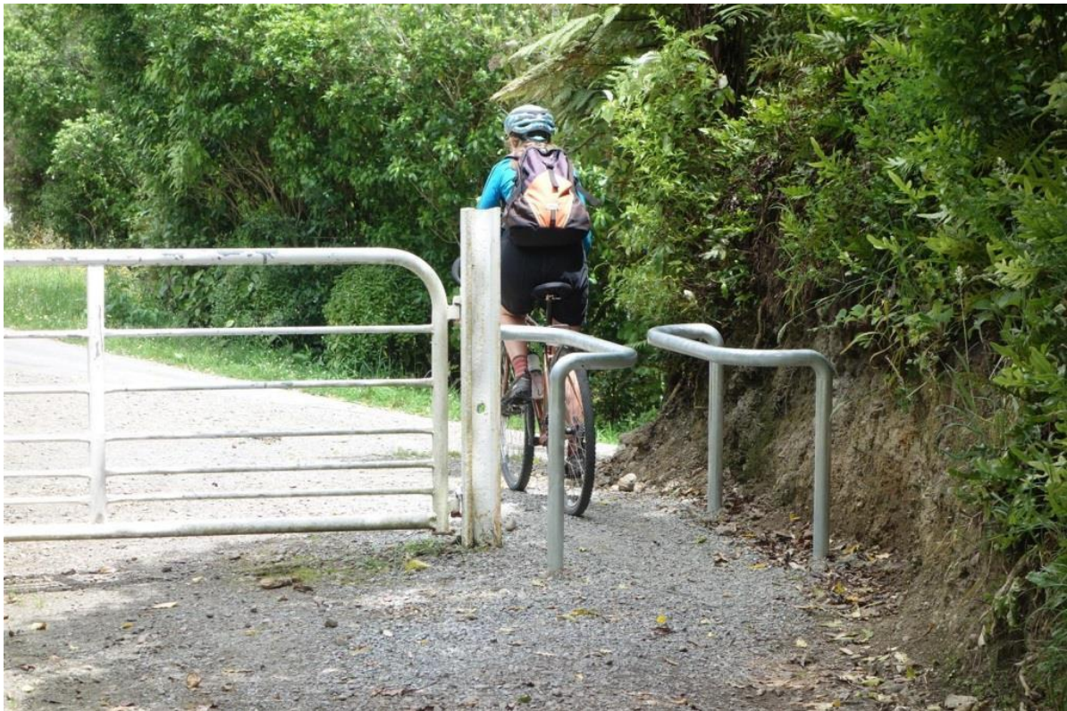
Figure E17: 'Squeeze barrier' to discourage motorcycles, Remutaka Cycle Trail (Photo: Jonathan Kennett)
