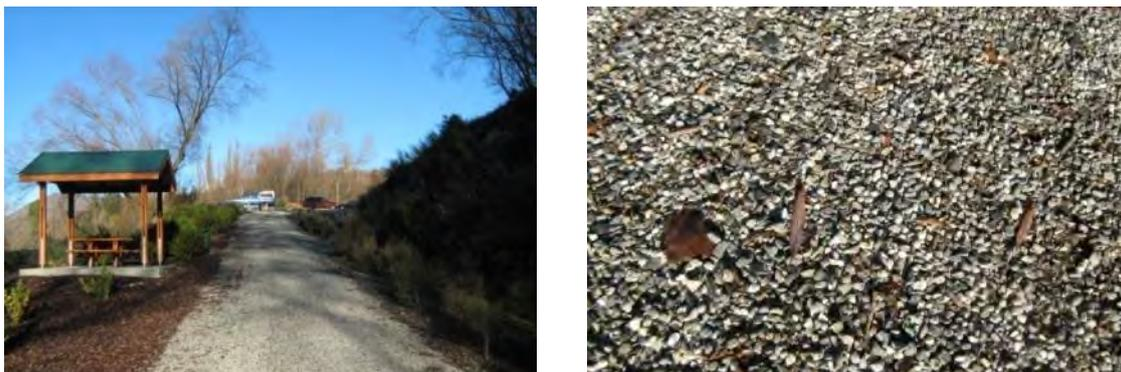
**Figure 24: Chip seal path in Queenstown**
