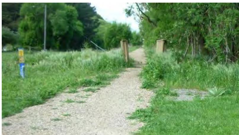
**Figure 20: Compacted gravel section of Little River Rail Trail at Catons Bay**
