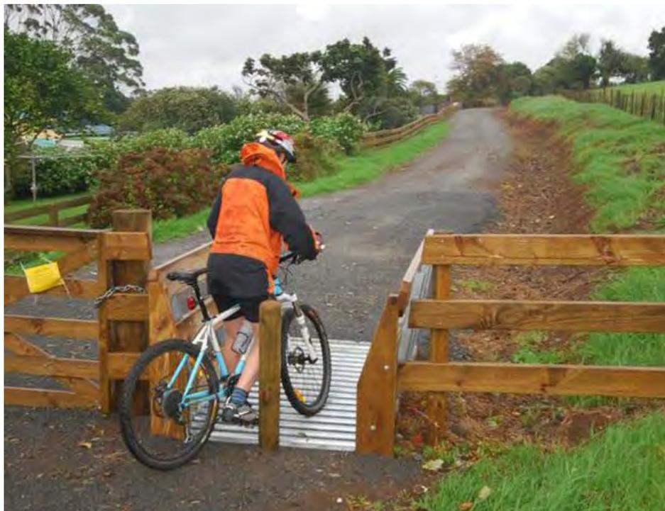
**Figure 59: A central post and wing barriers help prevent motor-cycle access and reduce the likelihood of stock jumping the cattle stop (photo Jonathan Kennett)**
