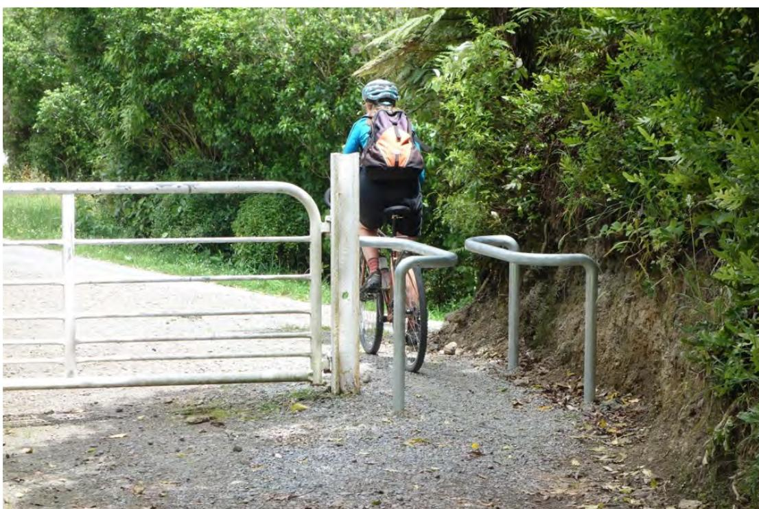
Figure 63: “Squeeze barrier” to discourage motorcycles, Rimutaka Cycle Trail (photo: Jonathan Kennett)
