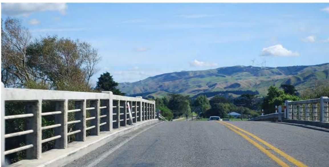
**Figure 48: Many railway overbridges have inadequate shoulder width and may require clip-on bridges on each side for cyclist safety (photo: Jonathan Kennett)**
