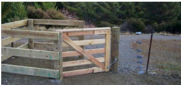
**Figure 60: Kissing gate: Hawea Track; can be difficult for tandems and bikes with trailers**
